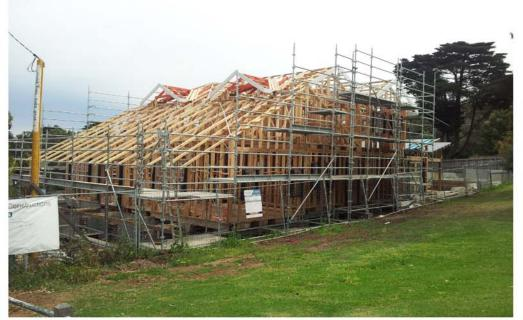
This job involved providing trusses to line up from lower level to upper level supported by a 12metre box girder running the width of the building, providing support for trusses & dormer's.
